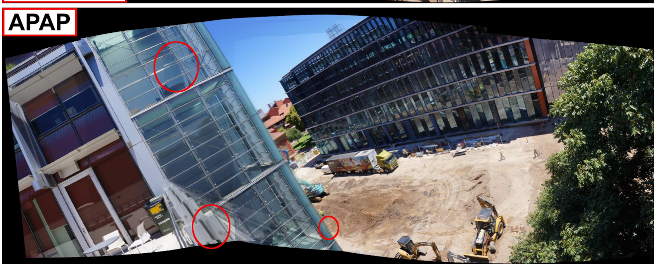
Fig. 9: Alignment results on the construction site image set (best viewed on screen). Red circles highlight errors. Note that photometric postprocessing was not applied on Autostitch and APAP.
